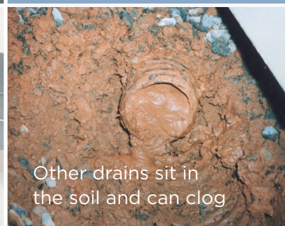
TYPICAL CLOGGED DRAINTILE
