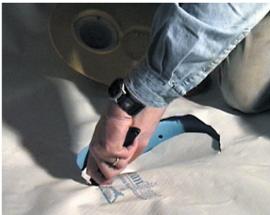
HOLE CUT IN CLEANSPEACE
